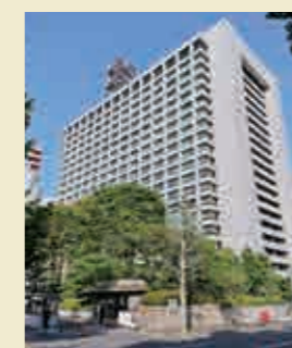
Central Gov't Bldg. No.2
