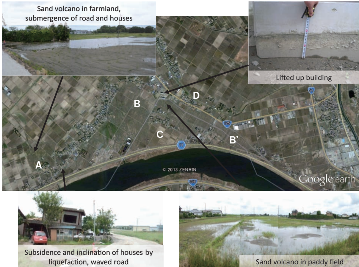
Fig.5 Liquefaction damage in Kessa and Kokuno area (base imagery by Google Earth), and ground photos in a field survey on 16th June, 2011
